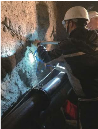
图3 传感器安装示意图 Fig.3 Diagram of sensor's installation
