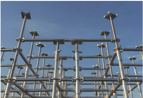
图 4 新型盘扣式钢管支架体系 Fig.4 New type of disk lock steel pipe scaffold system
