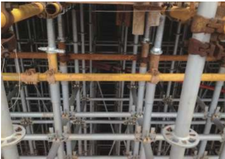
图 2 模板支架实景图 Fig.2 Real map of the steel pipe support formwork
